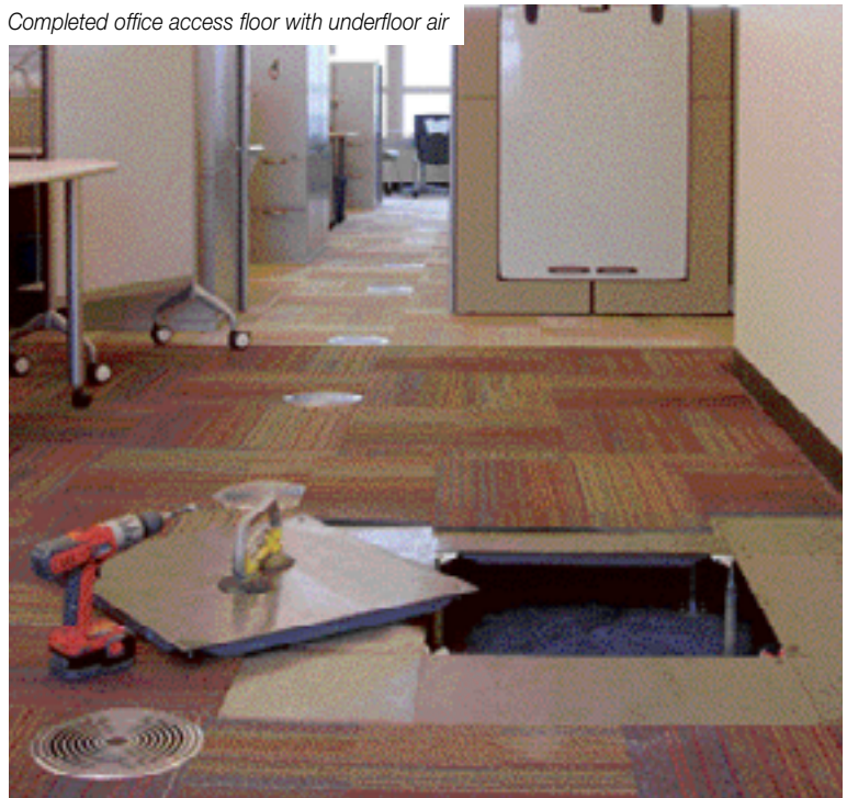
Completed office access floor with underfloor air
